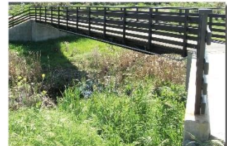
RAIL CAR BRIDGE CROSSINGS
